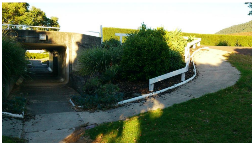
Figure 41: Vista Paku Underpass
