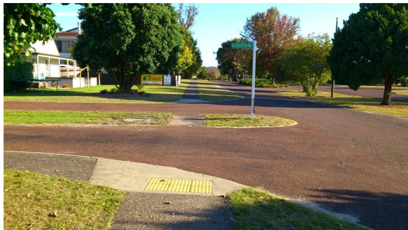
Figure 22: Tactiles at the Vista Paku/Coutts Road intersection
