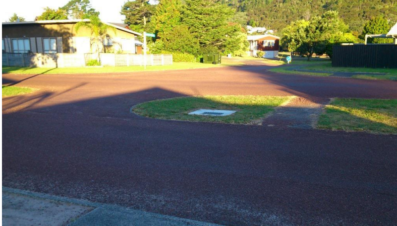
Figure 30: Crossing Pauanui Boulevard at Beaumont Green
