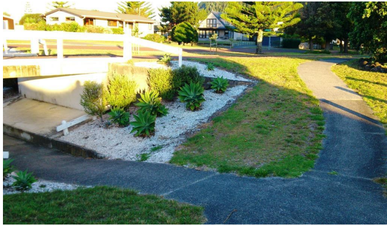
Figure 42: Underpass on Pauanui Boulevard
