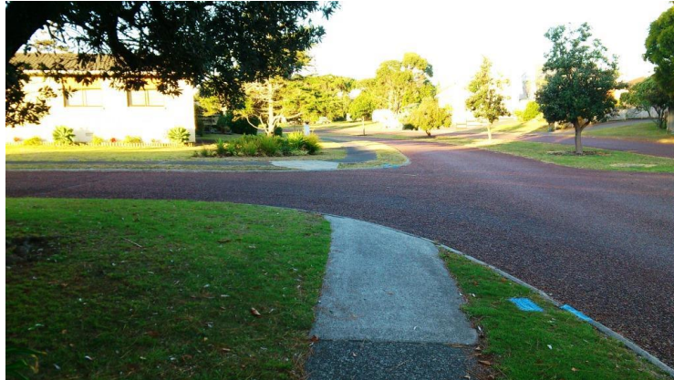
Figure 18: Kerb ramps at Britannia Dell
