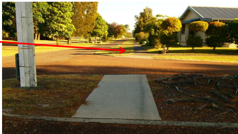
Figure 14: Alignment of crossing at the intersection of Vista Paku and Dunlop Drive
