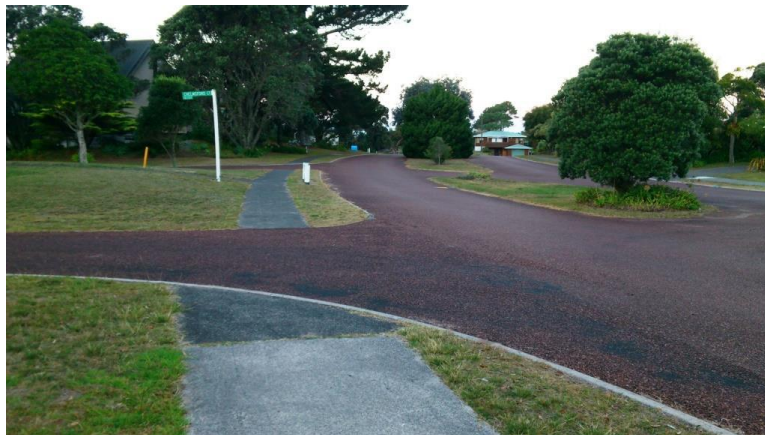
Figure 27: Jubilee Drive/Chelmsford Court
