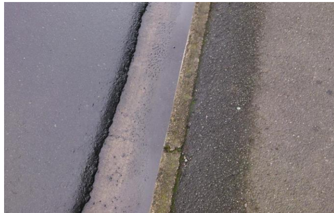
Figure 21: Seal edge join after re-sealing
