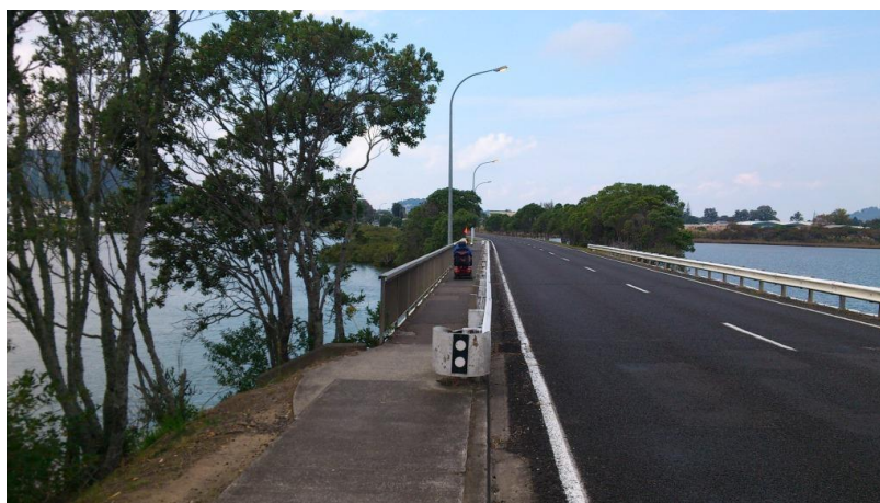
Figure 45: Bridge footpath on Harry Watt Drive
