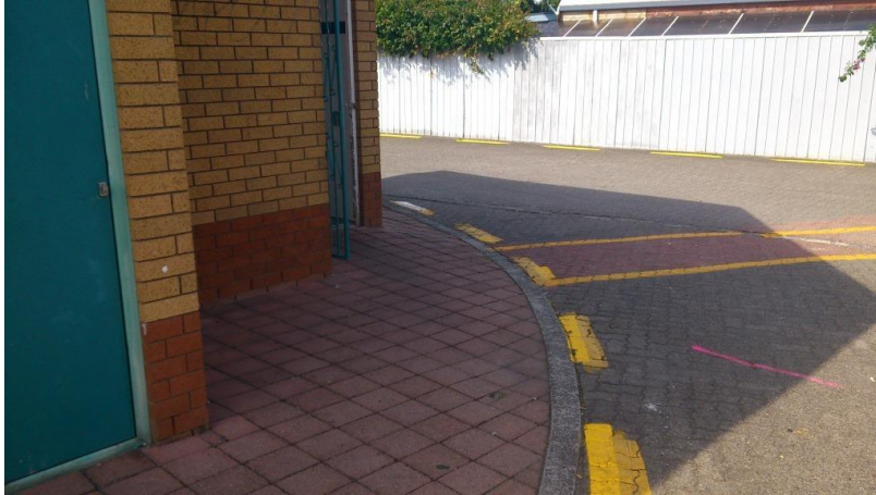
Figure 52: Walkway at Public Toilets near Port Road
