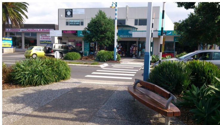
Figure 41: Light Poles on the wrong side of the pedestrian crossing on Port Road
