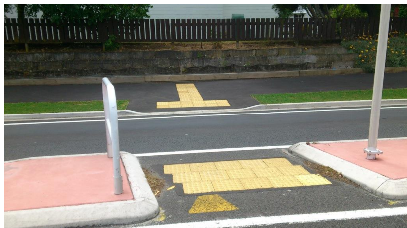
Figure 32: Ideal pedestrian refuge island crossing facility
