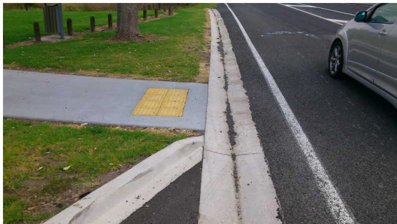
Figure 18: Tactiles on Hetherington Road
