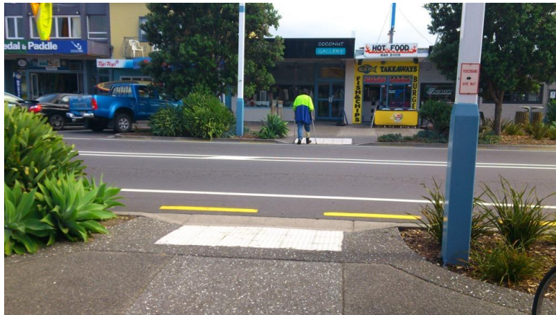
Figure 21: Tactile at a crossing point on Port Road
