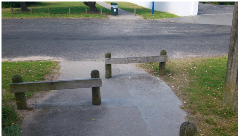
Figure 51: Chicane barrier at Mooloo Crescent
