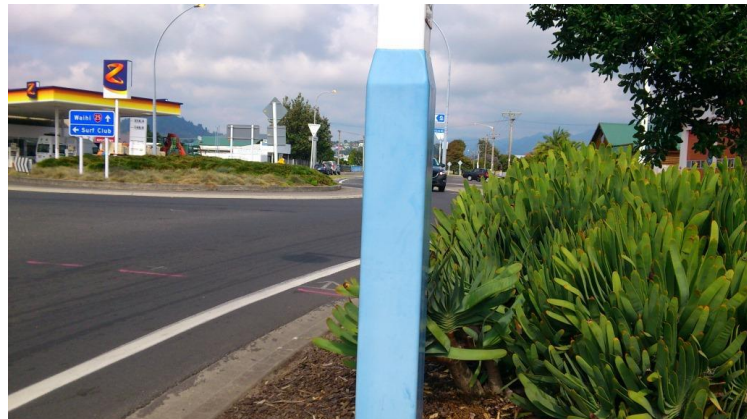
Figure 40: Light Pole affecting sight distance at Port Road/Ocean Road intersection
